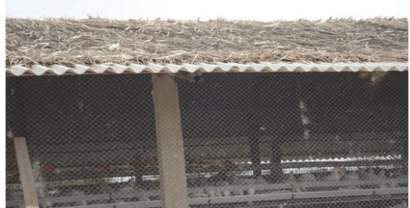
Fig 2: Effective use of thatching materials to reduce roof heating
