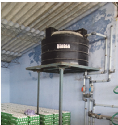
Figure 3. Water tank inside the shed keeps the water temperature cool.
