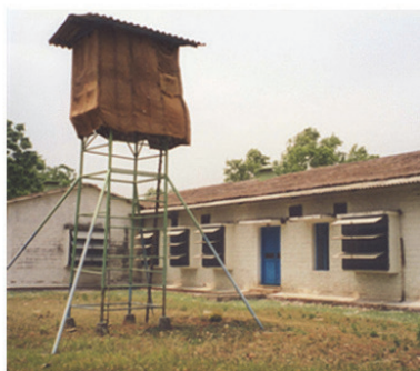
Figure 4. Outside water tanks should be white, insulated and covered to avoid direct sunlight.
