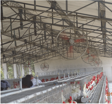
Figure 6. Shed using stir fans and foggers to reduce heat load.
