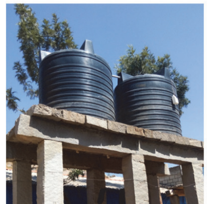
Figure 5. Water tanks should be covered to avoid excessive heating from the sun.
