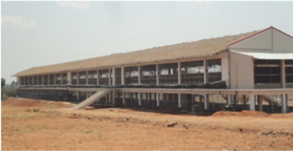
Fig 1: Roof thatching provides insulation to keep the shed cool
